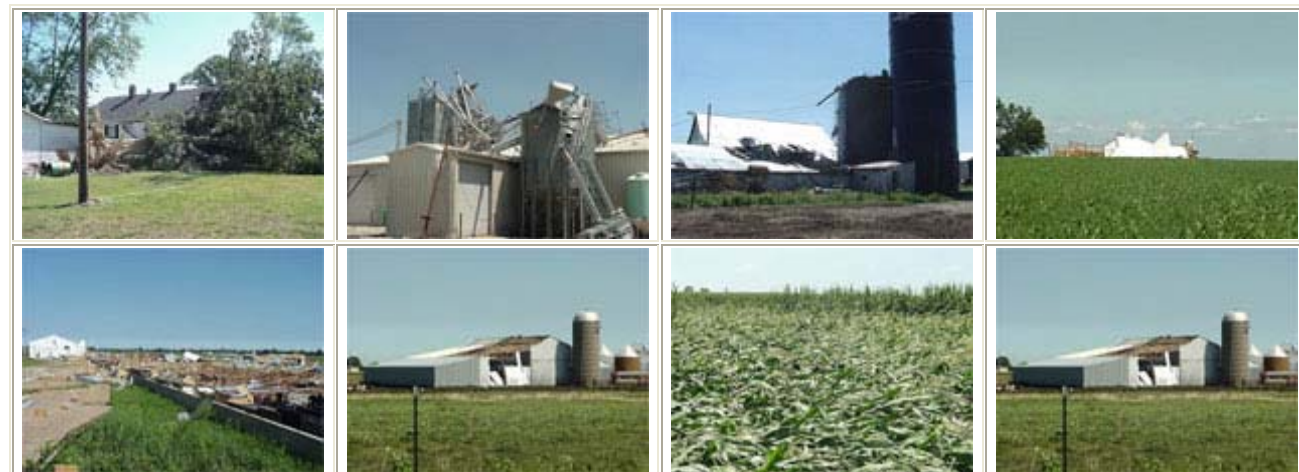
STORM DAMAGE PHOTOS FROM 21 JULY 2006
